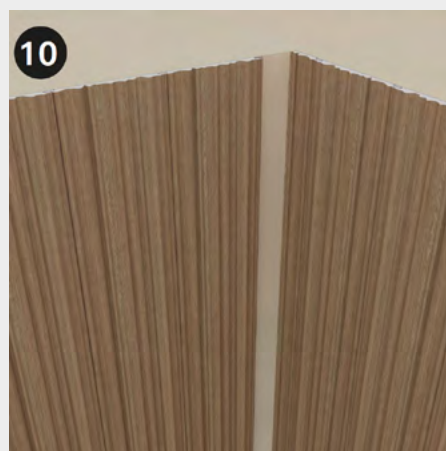
Install the panels on the other side of the wall in the same way as the previous ones. Measure the remaining space between the penultimate panel and the inside corner. Cut the panel according to the measurement obtained.
