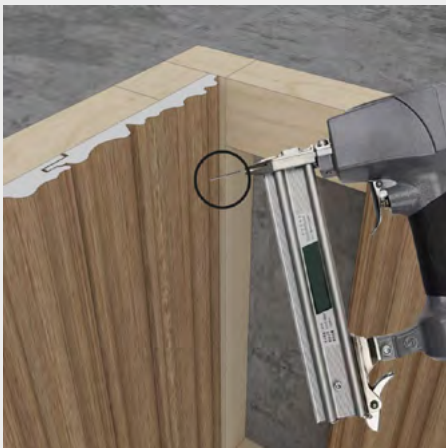
Install the cut panel by attaching it to the joints with the appropriate brads at a 45-degree angle.
