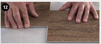
DISASSEMBLING SHORT SIDE Disassemble the row by sliding apart the planks on the short side.
