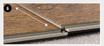
ENGAGE THIRD PLANK ON SHORT SIDE - 1 Using the patended lock system, drop the short side of plank 3 onto the short side of plank 1.
