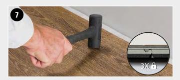
ENGAGE THIRD PLANK ON SHORT SIDE - 2 Using a soft-faced hammer slightly tap the joints on the short side to secure. This ensures 3x locking.
