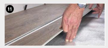
DISASSEMBLING LONG SIDE Wish to disassemble? Lift up the entire row, in the same angle as you did during installation, then slide apart the rows.
